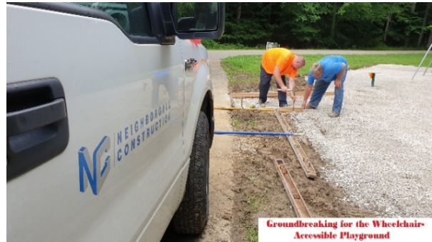
KSSF Installation of Adapted Playground
