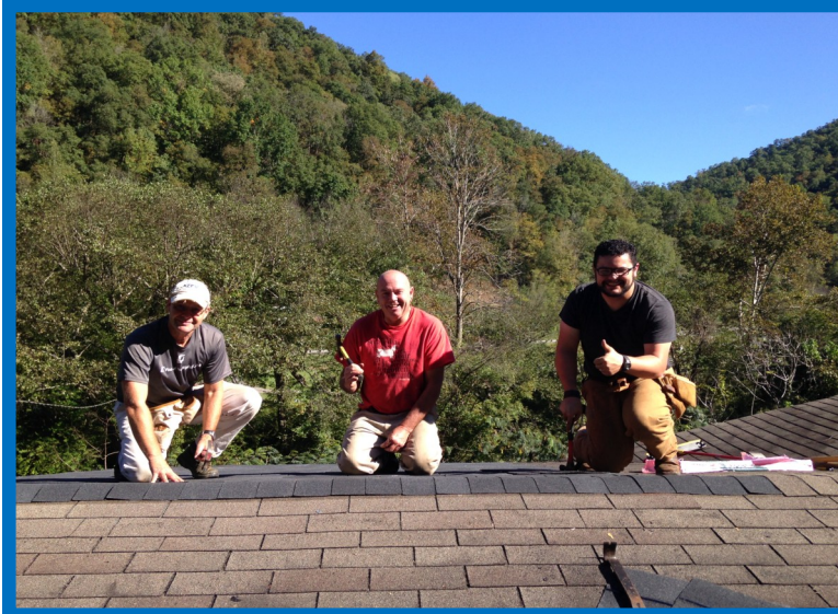
THE TROUTMAN BAPTIST TEAM REPLACE SHINGLES FOR A FAMILY IN MINGO COUNTY
