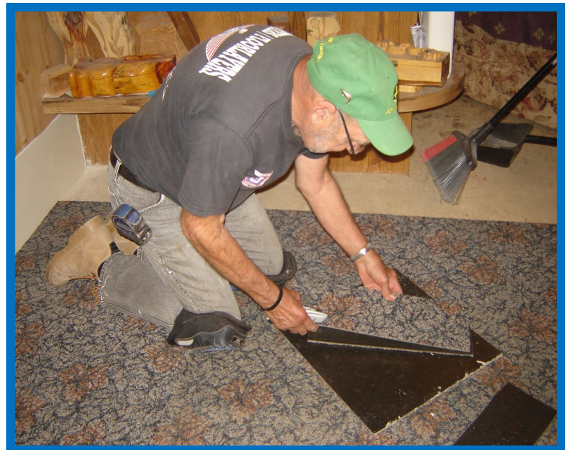
CARPET IS LAYED IN HOME DAMAGED BY FLOOD WATERS
