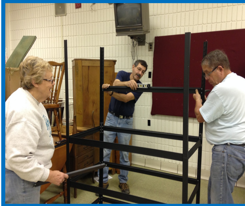
MEMBERS OF THE RICHFIELD UCC TEAM CONSTRUCT SHELVING FOR THE WAREHOUSE
