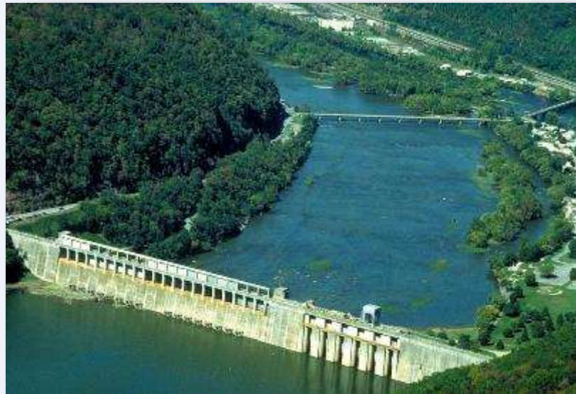
Bluestone Dam, West Virginia
